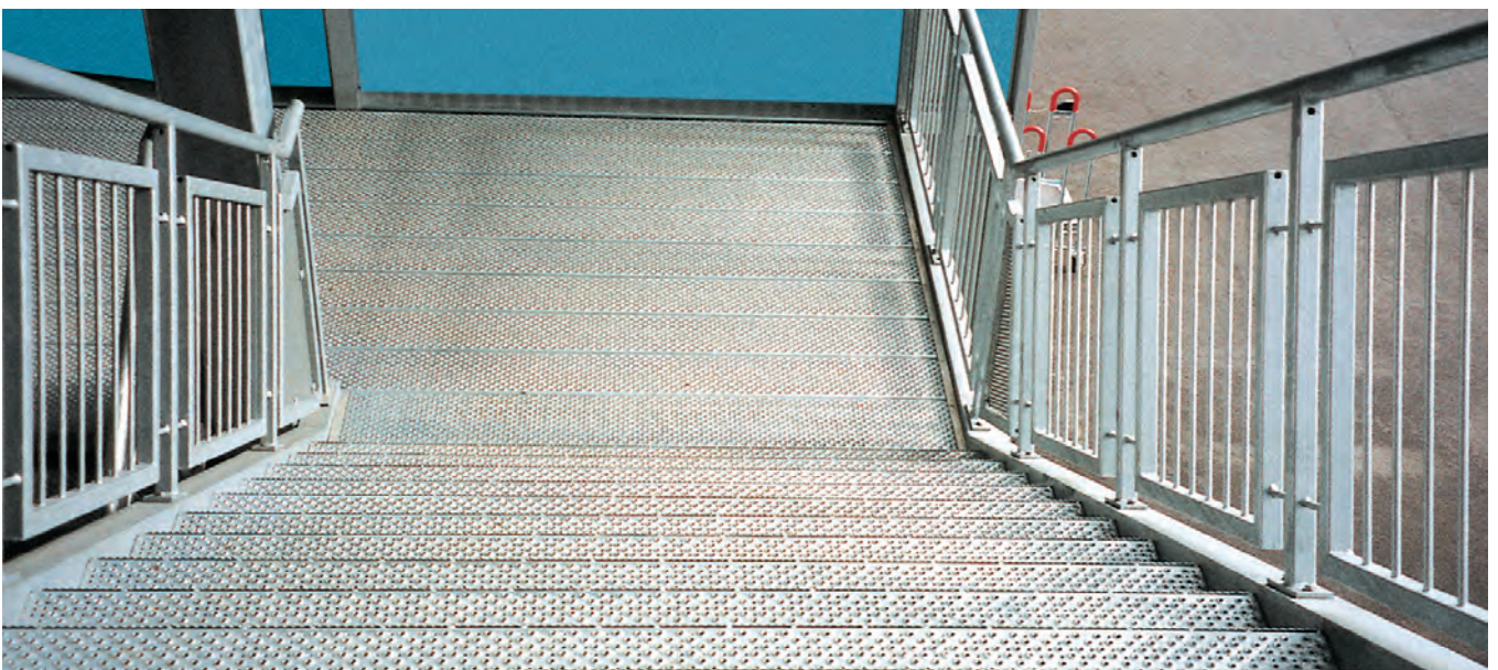
Staircase with intermediate landing
